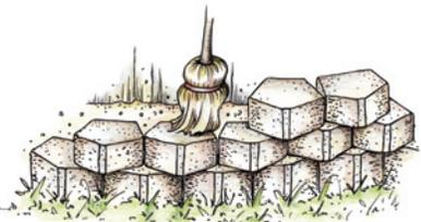
**STEP 4:** Continue leveling from side-to-side and front-to-back, compact loose dirt behind the wall.
