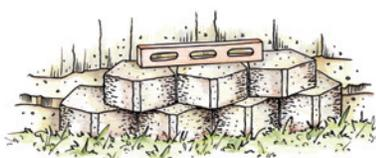
**STEP 3:** Position next course of block on top of the first, utilizing the cross bond pattern.
